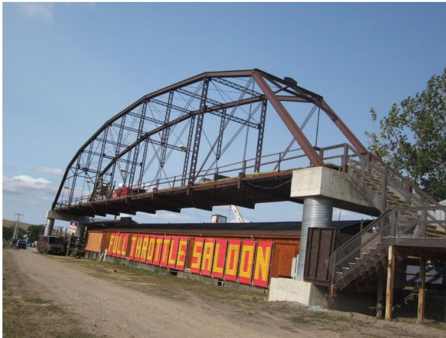
Figure 6. Example of a change in the character of a property's use and of physical features within the property's setting that contribute to its historic significance. The bridge is no longer used for its intended purpose, and the setting of the bridge has been entirely altered by moving the bridge to a new location.
