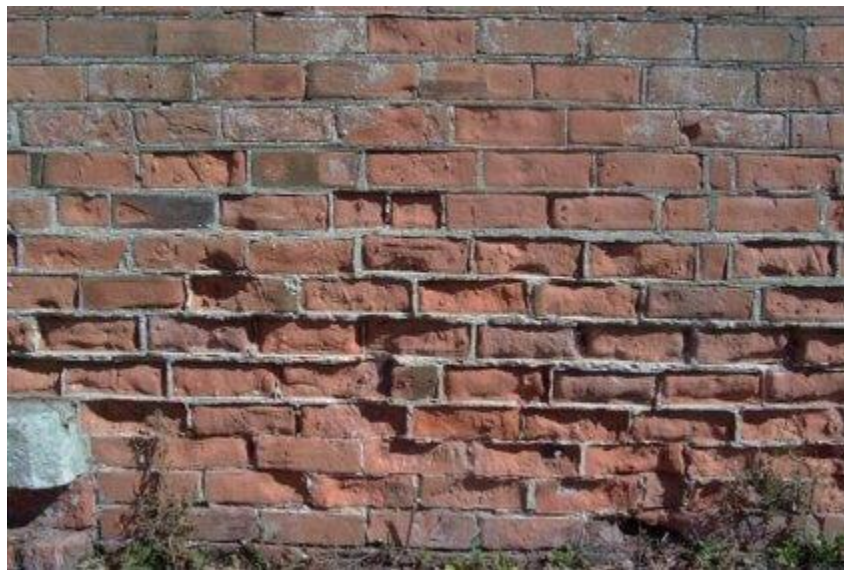
Figure 4. Examples of alterations to properties which are not consistent with the Secretary of the Interior's Standards for the Treatment of Historic Properties. In the top photographs, enclosing the porch caused drastic changes to the house's historic character. In the bottom photograph, repointing with inappropriate mortar forced moisture through the wall, eventually causing the brick to spall, crack, and disintegrate. The latter is an example of an adverse effect that can occur later in time.
